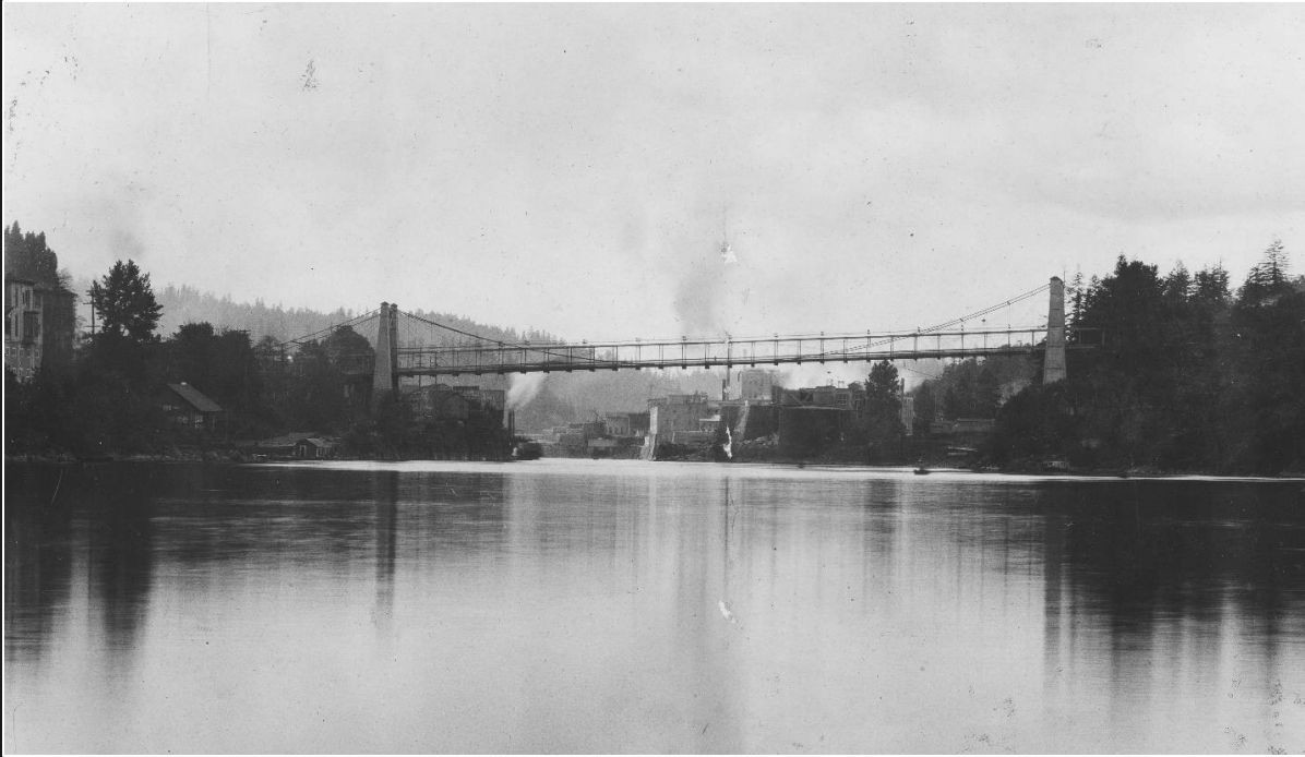
Looking upriver at the Willamette River Bridge at Oregon City, which opened in 1888.
