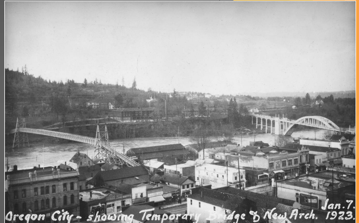
Photo showing temporary bridge upstream of the new Willamette River (Oregon City) Bridge shortly before being dismantled in 1923.
