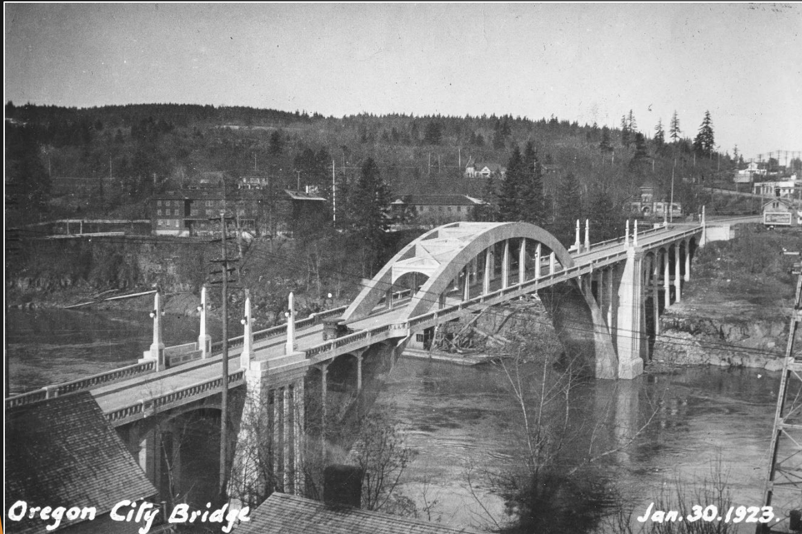
Willamette River (Oregon City) Bridge shortly after dedication in December 1922.
